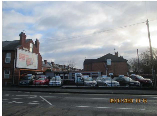
View of north west boundary and side elevation of no. 1 Hawthorn Grove on right and side elevation of no. 145 on left
